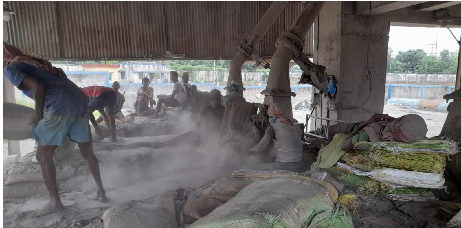
Ash Bagging System
