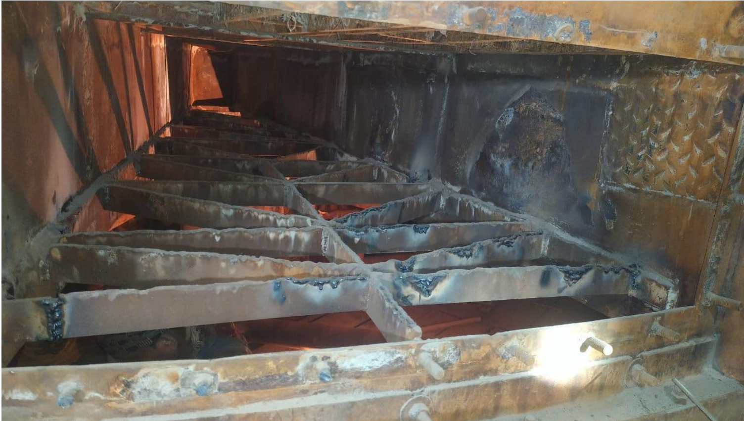
AIR PRE-HEATER OVERHAULING JOB
