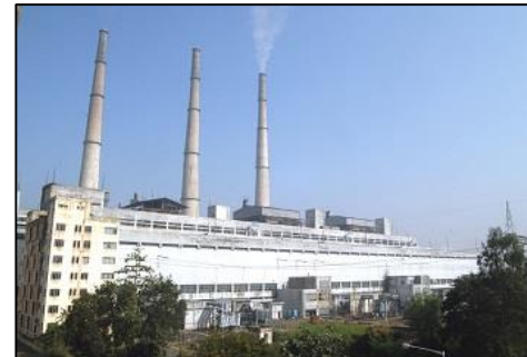
KOLAGHAT THERMAL POWER STATION(KTPS) TOTAL CAPACITY: 6X210MW
