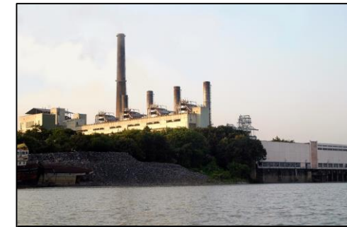
BANDEL THERMAL POWER STATION(BTPS) TOTAL CAPACITY: 2X600MW, 1X215MW
